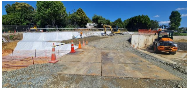
“Luke’s Bridge” set up for machinery movement over the pipe
