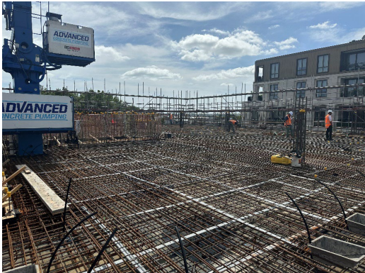
Level 2 area B steel reinforcement, progress on rebar foundation
