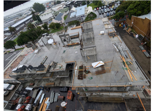
Building R – Suspended slab level 3
